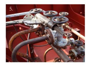
6. By chipping it is very clear, that piping locally suffers from heavy corrosion.
