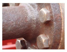
8. Wencon Cleaner applied with a brush, to degrease pipings, prior to application.
