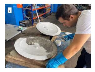
3. & 4. First layer of Wencon Coating applied with a brush, in layer of 500 microns. Then left for semi curing in approx 1 ½ hour.
