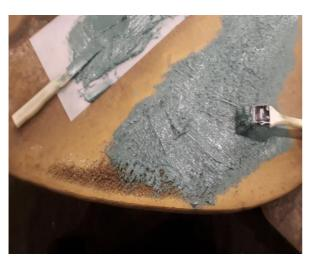
8. To optimize adhesion, the 1<sup>st</sup> layer Wencon Ceramic Cream are "worked toughly" into all pores and unevenness of the cavitated arias.
