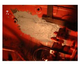
8. Curing was allowed, with an additional 1000W lamp to heat it a little up, because of the low temperature.
