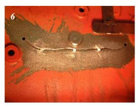
7. 3 layers of Wencon Rapid were applied. The first one a thin layer and then a piece of Reinforcement Tape in the layer. Next, 2 layers of Wencon Rapid were applied on top, with Reinforcement Tape between.
