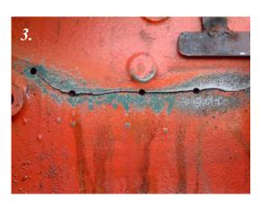
4. Self-tapping screws were placed in each hole, except for the two extremes positions, to prevent the crack from moving.
