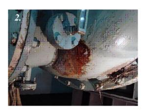
A small spot slowly dripping was discovered after ended application. Presumably caused by pressure on the end cover from the inside. Wencon recommended to add some extra layers of Wencon UW Cream on top, to stop the leakage completely.
