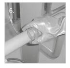
6. If the pipe cannot be emptied, use the Wencon Putty. Eventually hold it in place with a small metal plate and a steel band, before applying the pipe tape.
