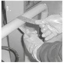
1. Empty and clean the leaking pipe and grind it with emery paper or the like.
