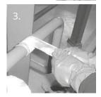
3. Wrap the Wencon Pipe Tape tight around the pipe. (min. 9 circles)
