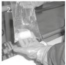
2. Unpack the Wencon Pipe Tape and submerge it in water for 30-40 seconds. For higher pressure, use Wencon Putty. (se fig. 6)
