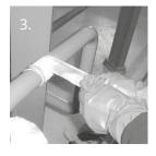
3. Wrap the Wencon Pipe Tape tight around the pipe (min. 9 circles), with 50% overlap, extending 50 mm beyond the damage.
